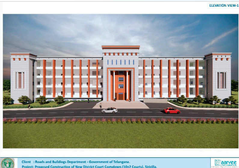
Client : Roads and Buildings Department - Government of Telangana. Project: Proposed Construction of New District Court Complex (192 Courts), Sirilla.
